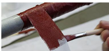
**11.**▶ At the end of the second layer cover the upper and lower side of the fabric tape with sealing compound.
