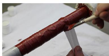
1. ▶ Mask the area which will be sealed with a suitable adhesive tape (e.g. Tesa tape, crepe tape)
