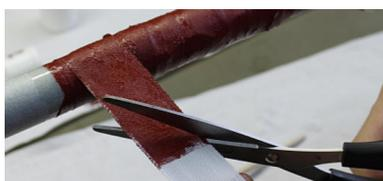
**12.**▶ Cut the fabric tape with scissors diagonally.
