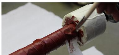
**10.**▶ Without interruption add a further layer of fabric tape and fix it with sealing compound.
